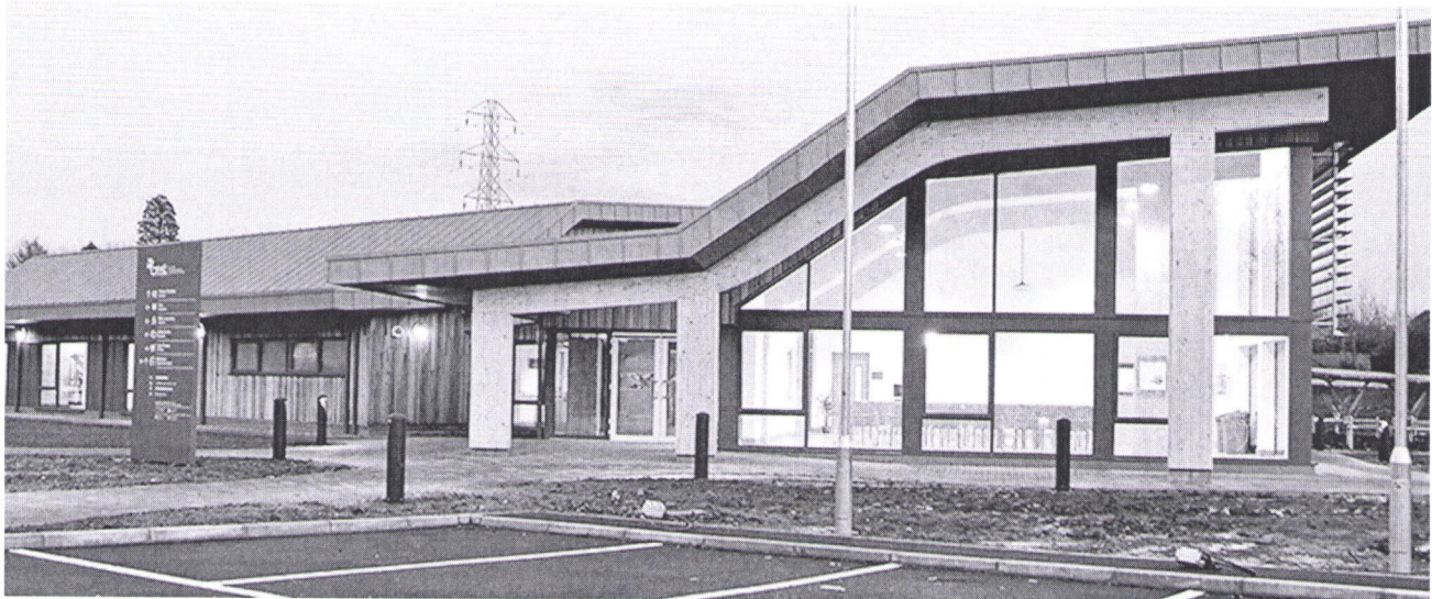
Figure 1: The CREST Pavilion with design featured solar control in brise-soleil and large overhangs.
